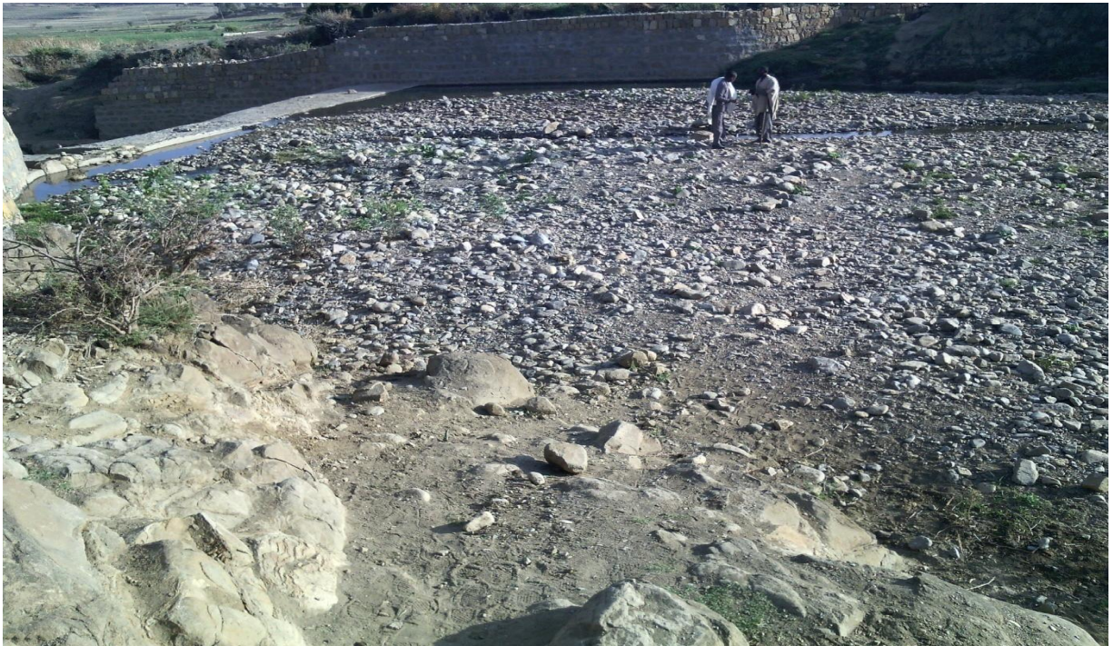
Appendix.Figure 5: At the upper of Gereb-segen the diversion silted at one year after construction
