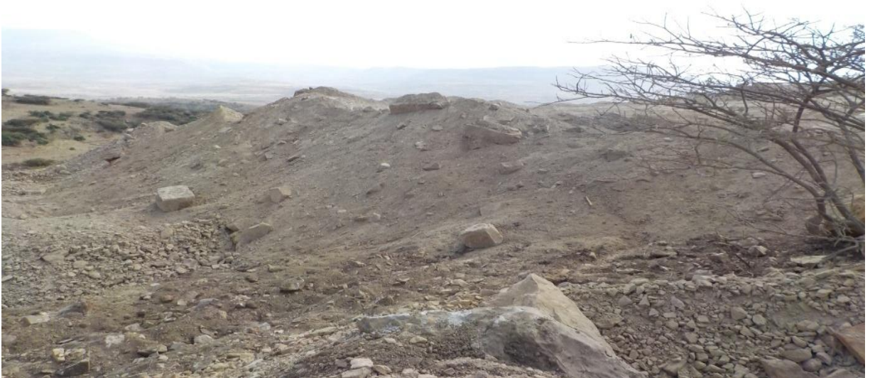
Appendix.Figure 7: Removal of bushes and disposal of soil at the upper Gereb-segen dam reservoir
