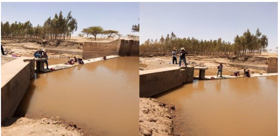
Figure 3.6: Headwork in Furfuro Irrigation Scheme
