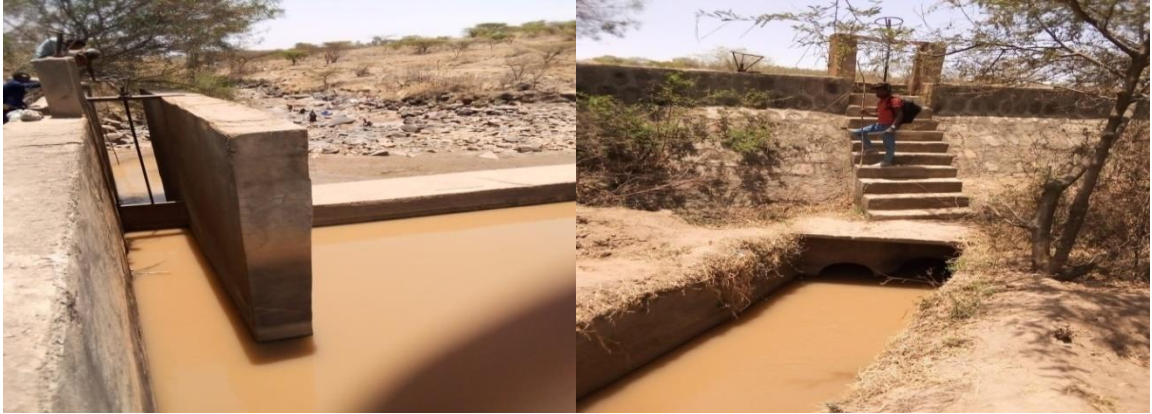
Figure 3.4: Headwork and Head Regulator in Bilate Irrigation Scheme
