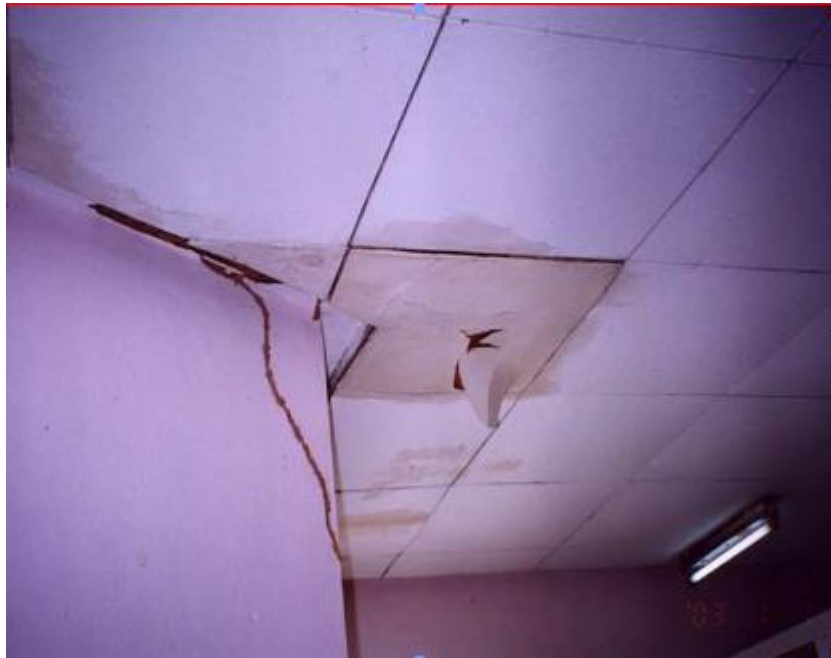
Figure 2.7 Ceiling moisturizing (James & Ransom, 2006).
