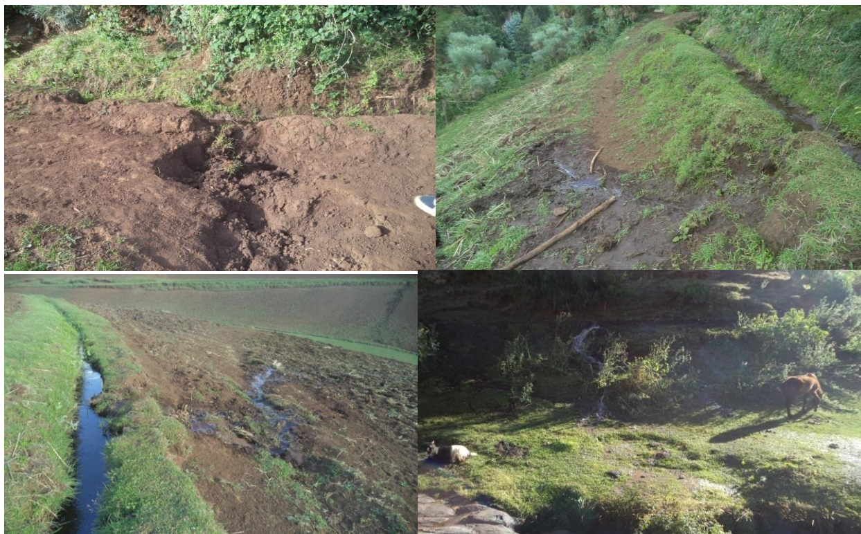
Figure 3 some of distorted canals alignment
