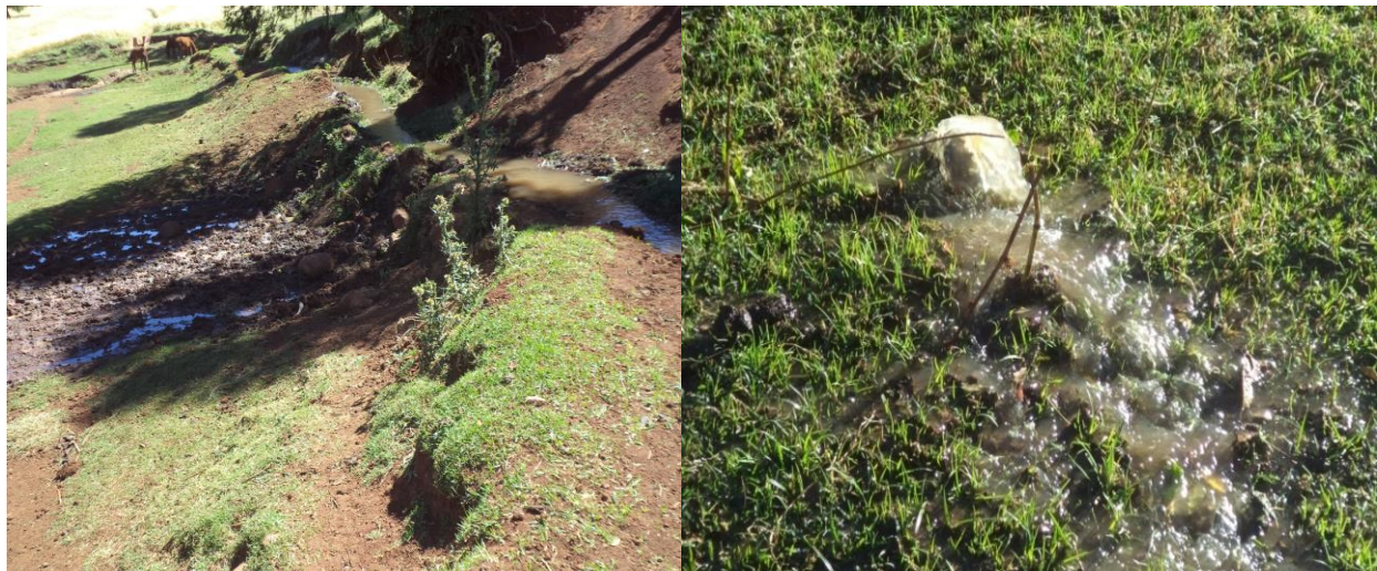
Figure 4.4 Canal water loss occurs at Gusha Elasa
