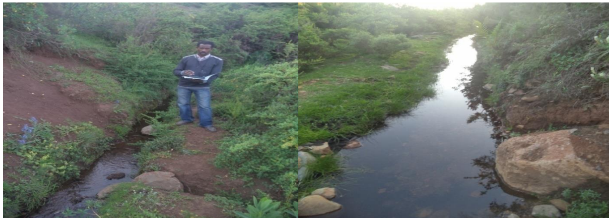
Figure 4.2 Main canals and head work of Gusha Elasa irrigation system.
