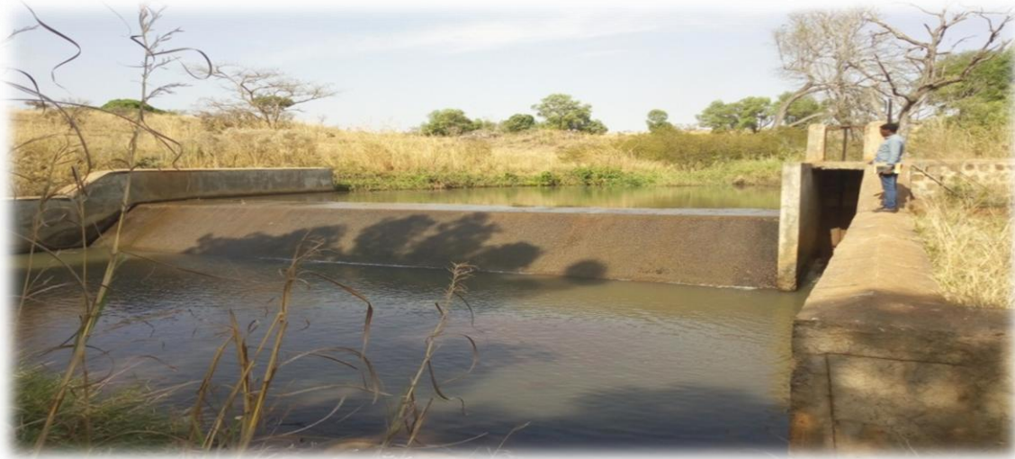
Figure 2.2: Diversion Weir of Golda irrigation scheme
