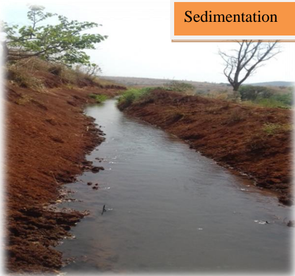
Appendix 2.4 : Low water level in the main canal due to sedimentation, un-clean grass, seepage and erosion
