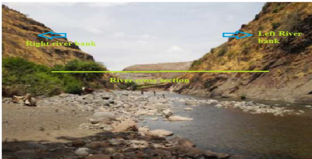
Figure 3. 4: Picture of propose dam site at alternative site
