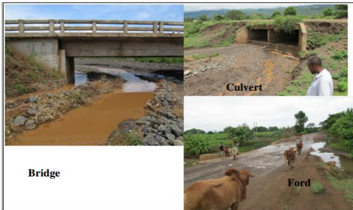
Figure 2.1: Primary drainage infrastructure types
