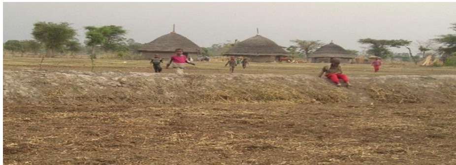
Figure 3.9: Flood Protection Structure on Guricho Kebele (Source Author)
