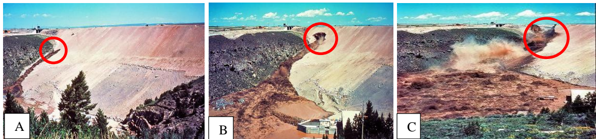
Figure 2-2: Sequential image of Teton dam piping scenario
