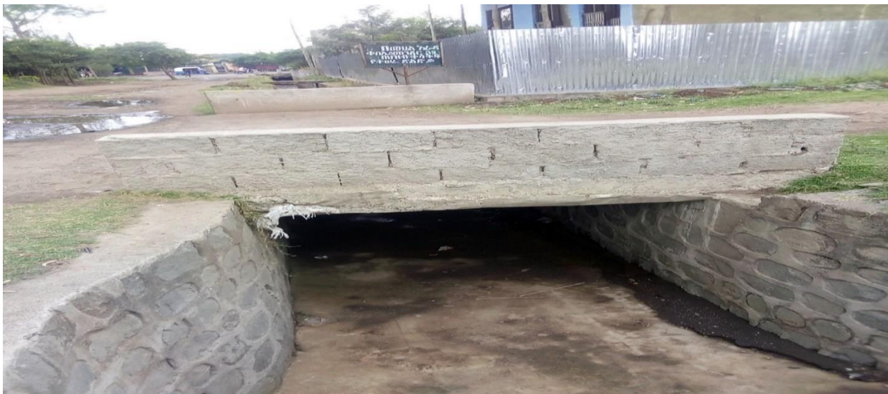
Figure C1: Manning's coefficient ( n = 0.020 (lower) and 0.015 (upper) are taken
