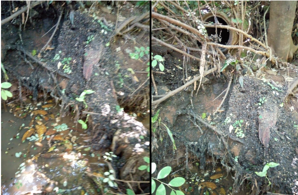
Figure a 5: Constructed pipes to discharge effluent and its effect on Chichu River quality
