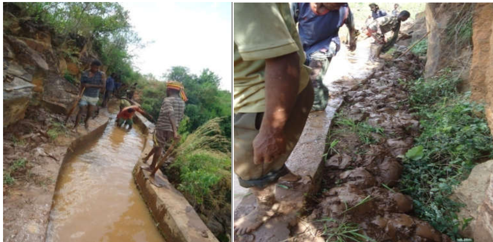
Fig-10, Silt excavation from canals in Litala irrigation scheme
