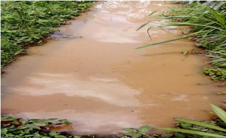
Appendix figure7: Evident of buried canal segments covered by weeds and soils
