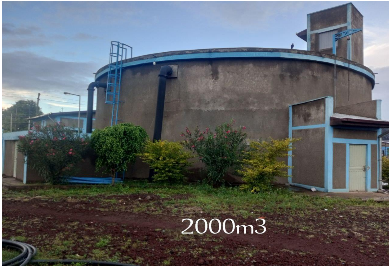
Figure 3 3: The existing 2000m3 reservoirs in the town
