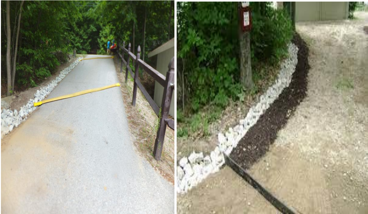
a) Asphalt road
