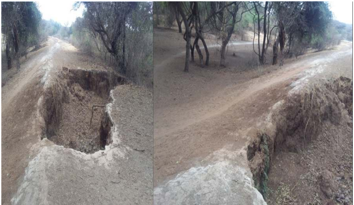
Figure 27 locally made earthen dyke
