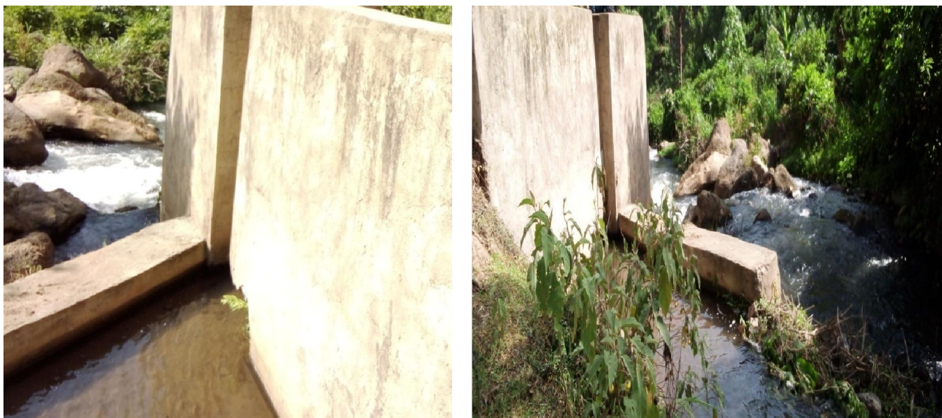
Figure 2: Wesha SSIS diversion weir structure
