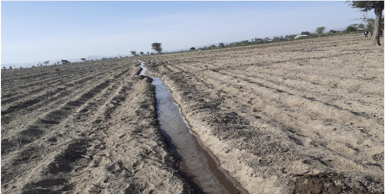
Figure 4. 5: Main canal before it is covered with plastic membrane
