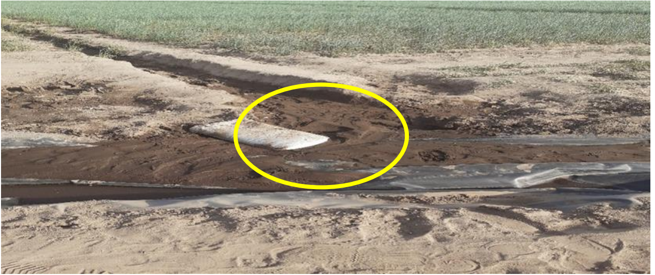
Figure4. 7: Sediment accumulation in main canal
