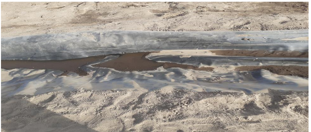
Figure 4. 5: Main canal before it is covered with plastic membrane
