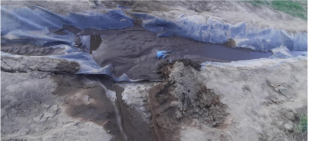
Figure 4: Sediment accumulation in canal
