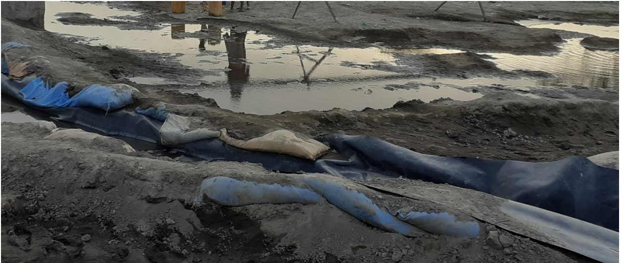
Figure 4: Sediment accumulation in canal
